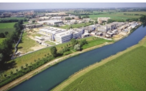
Settala's plant overview
