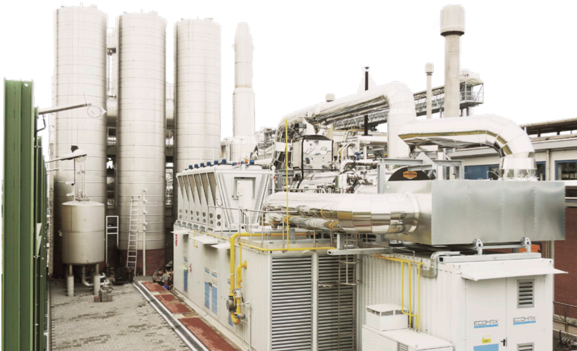
Settala Site Cogeneration plant
